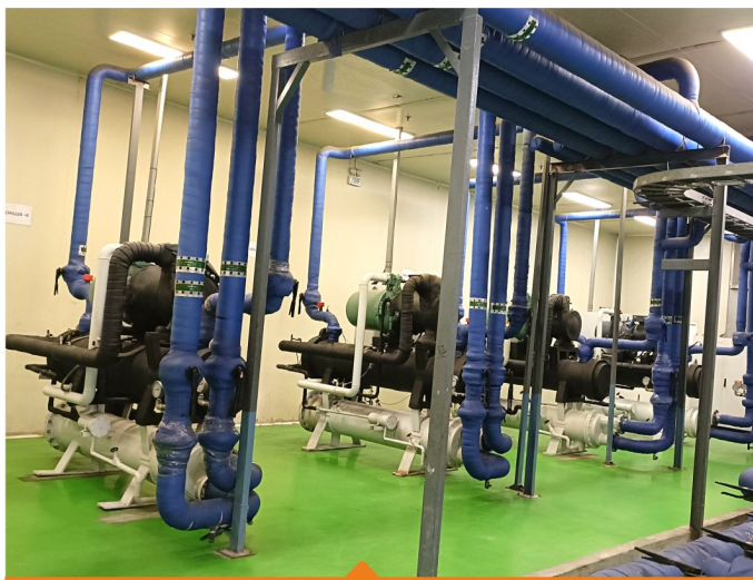
SCREW CHILLER INSTALLATION IN A MOBILE MANUFACTURING PLANT
