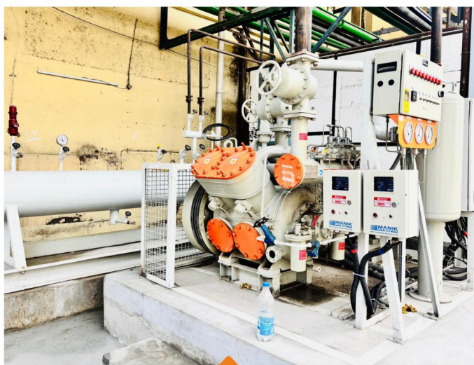
AMMONIA CHILLER INSTALLATION IN A DISTILLERY PLANT
