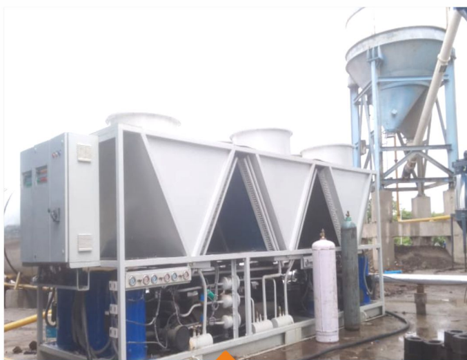
BATCHING CHILLER INSTALLATION AT CONSTRUCTION SITE
